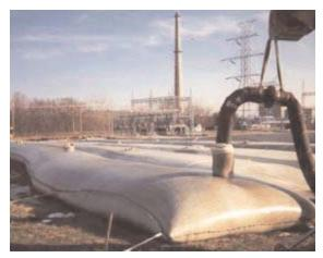
Figure 15. Geotextile tubes.
